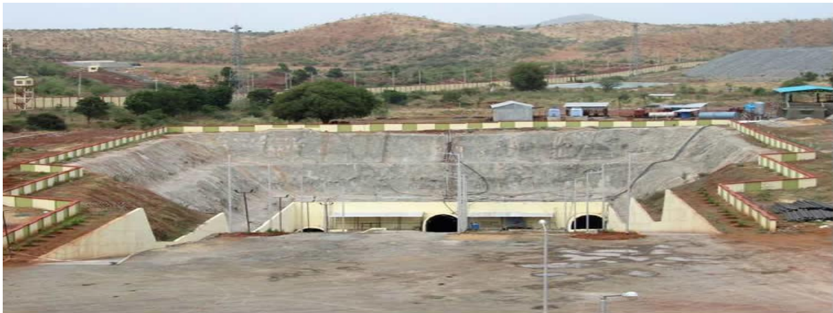
Photograph AIR INLET AND ENTRENCE TO THE MINE
