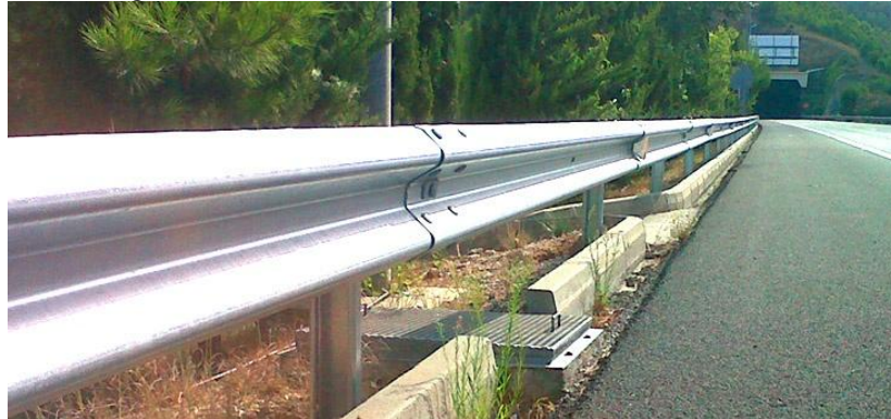
Fig3: View of Metal Barrier
