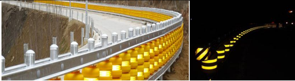
Fig5: View of installed Rolling Barrier in Curved Path both in day light and night reflection system
