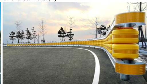
Fig2: View of installed Rolling Barrier
