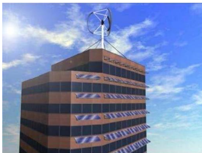
Fig. 2. Wind and PV-based power generation for the vertically integrated microgrid.
