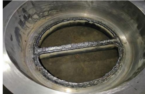
Fig 3- Dual plate check valve after welding
